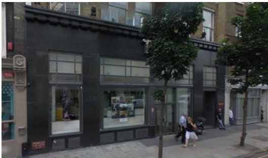
Image 17: Pre-Existing Shopfront Circa 2008
